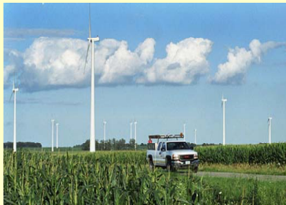
Wind farm a few miles west of Mason City, IA. Wind farms are scattered throughout northern Iowa and are a great source of energy (Wind Power Photo Gallery)
